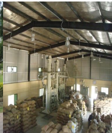
Seed processing plant
